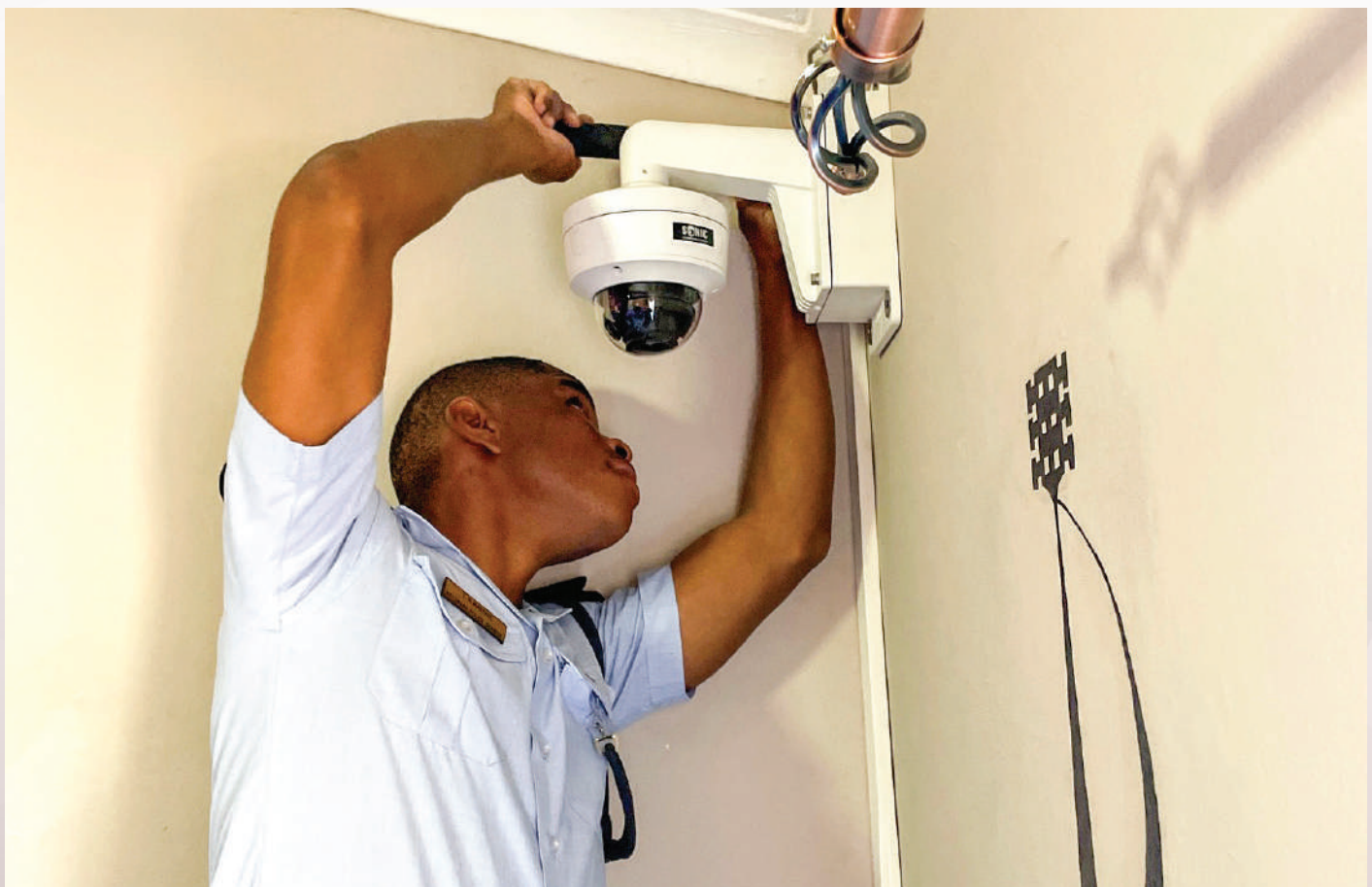
A police officer installing a CCTV camera in one of the police buildings
